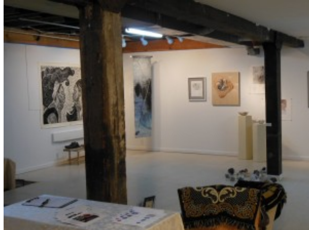
Wooden post and beam construction is evident in the converted arabber stable. (Anthony C. Hayes)
